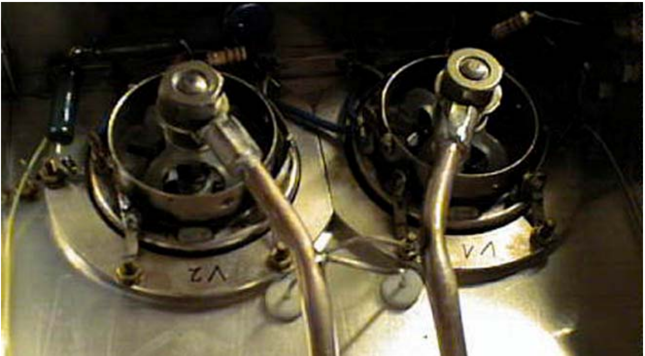
Close up of valve sockets and neutralising capacitors
